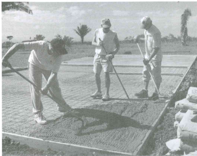
Pouring concrete for the classrooms.
