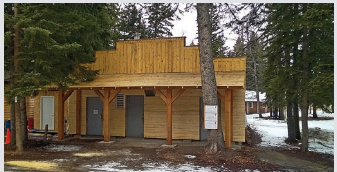
Foothills Camp New Washroom Block.
